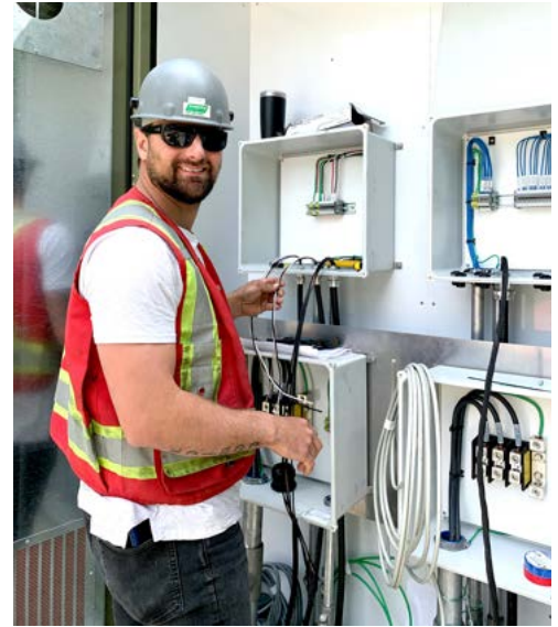
Emery electrician Kyle C. working on the Residual Solids Conveyance Line
