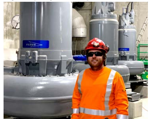
Ryan B. working at Macaulay Point Pump Station
