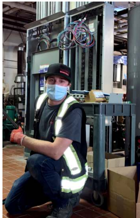
Brother Tyler working on fire suppression upgrades
