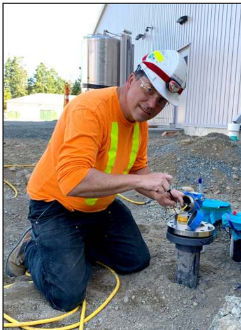
Brother Ken P. working at the Parkville Water Treatment Plant
