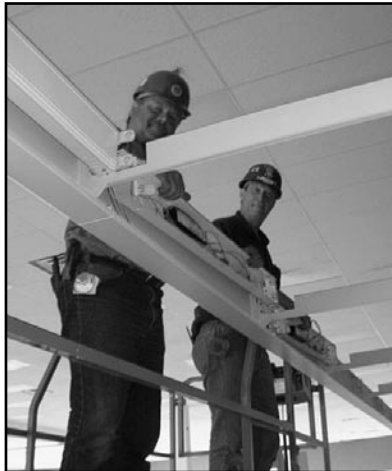
Brothers R. Farnsworth & K. Copping install fluorescent fixture strips.
